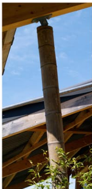
DETAIL PILIER BAMBOU
